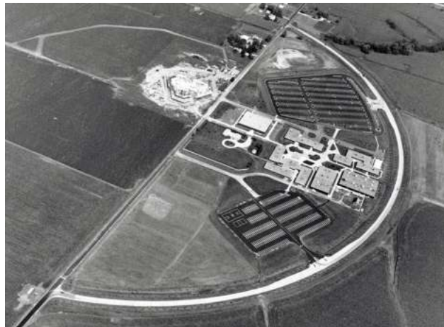
Original six one-story buildings and Brookens Library under construction in the early 1970's. Photo courtesy of www.uis.edu
