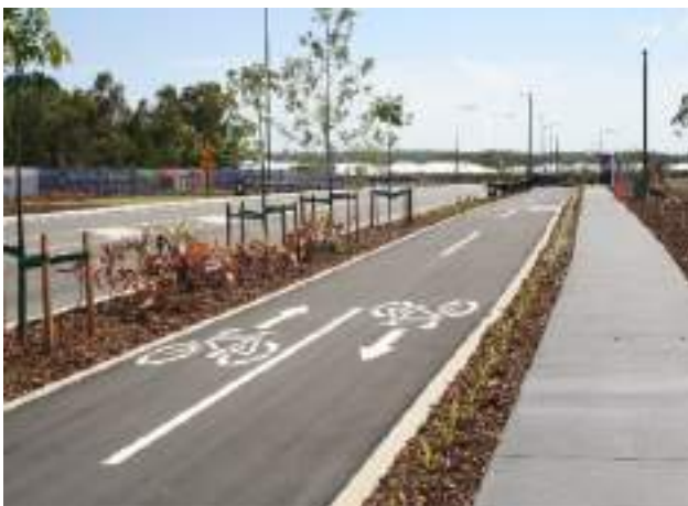
Raised two-way cycle track and sidewalk Photo courtesy of Kimley-Horn.
