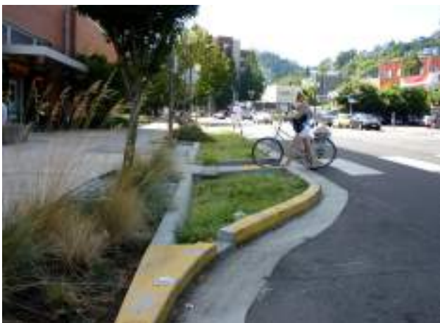
Curb extension located at mid-block pedestrian crossing. Photo courtesy of NACTO via Kimley-Horn.
