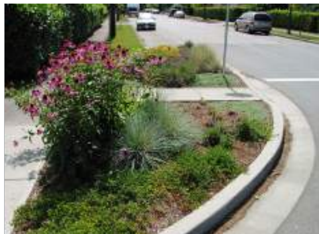
Curb extension located at intersection. Photo courtesy of NACTO via Kimley-Horn.
